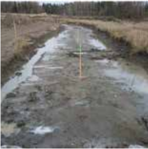
MUNICIPAL UTILITY WORK
