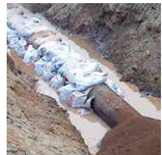
PIPE LINE WORKS
